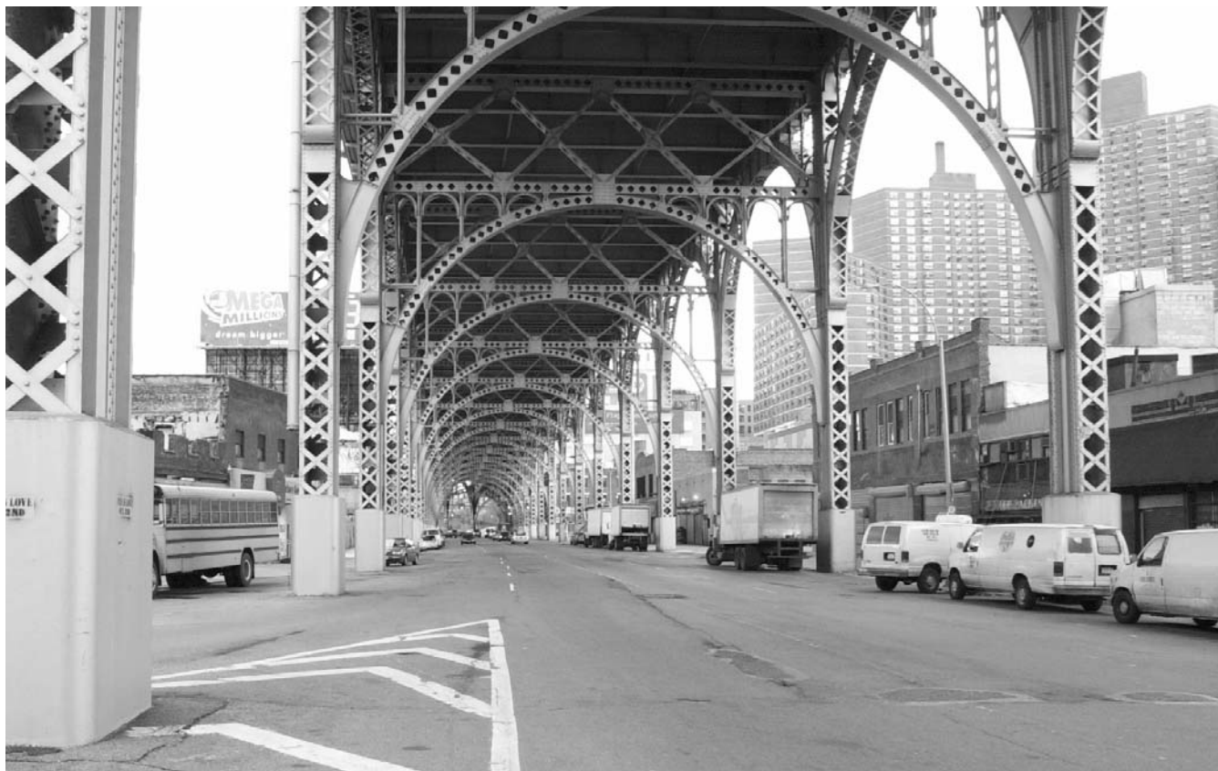
Viaduct near Harlem Piers. Businesses here could be affected by the Columbia expansion and the mayor's waste plan.
